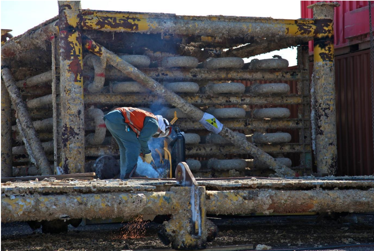
Disassembling a sub sea heat exchanger for decontamination
