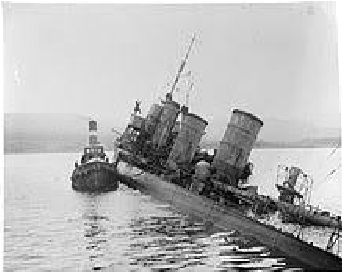
Kaiserin successfully raised, her eight air-locks secured by a web of guy-wires. (Fox Photos)
