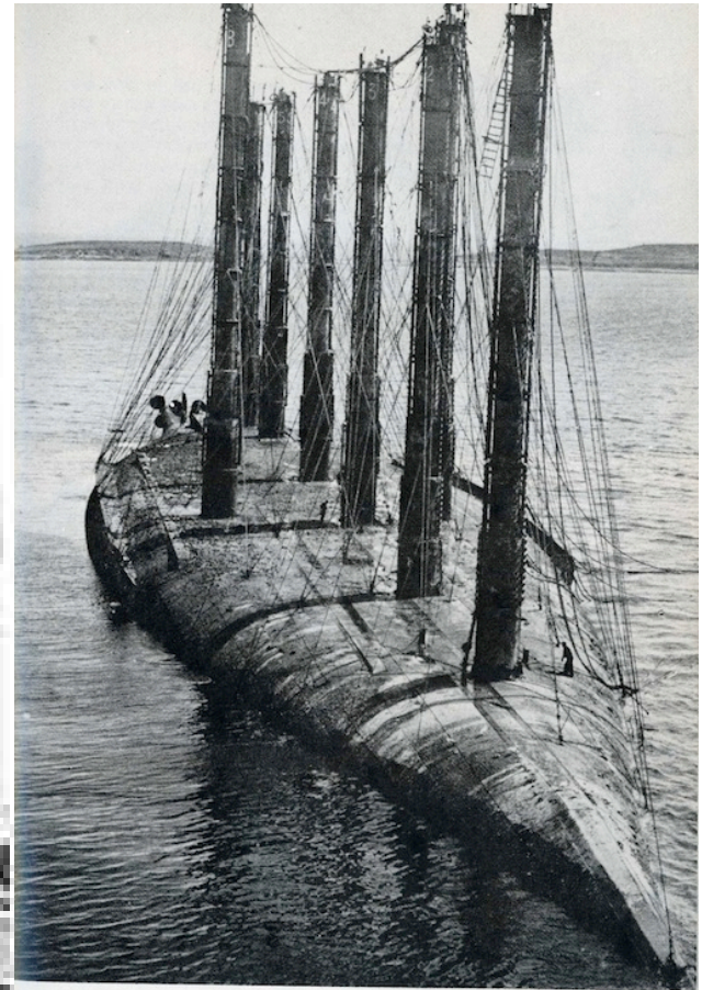
Kaiserin successfully raised, her eight air-locks secured by a web of guy-wires. (Fox Photos)
