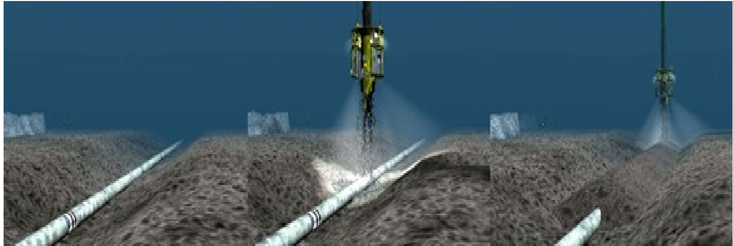
Trenched pipelines during rock burial
