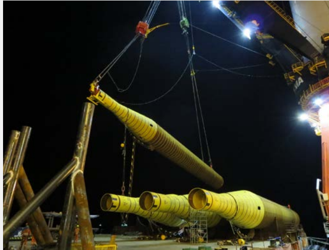
Lifting from barge
