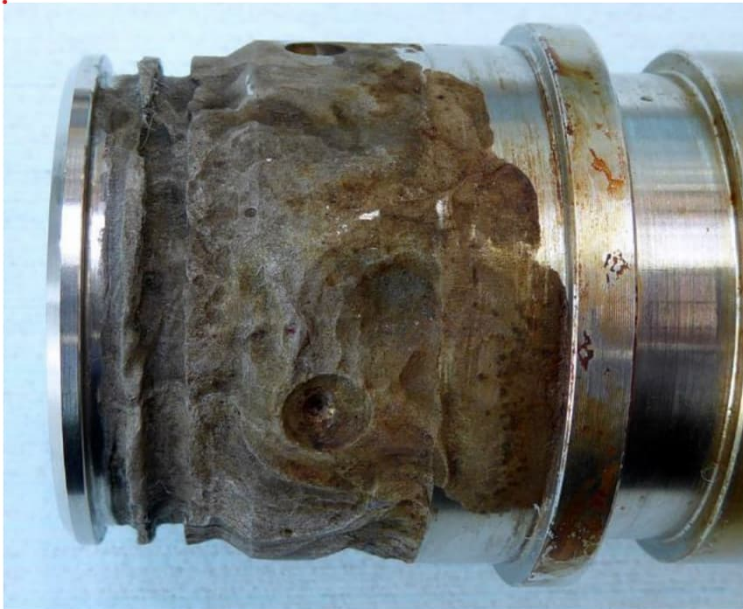
Figure 26 – Corrosion to plug body
