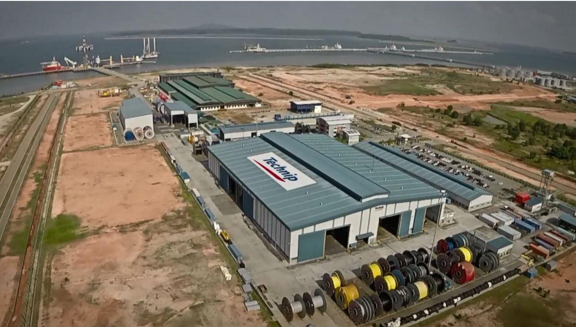
Figure 33 – AsiaFlex Manufacturing Unit
