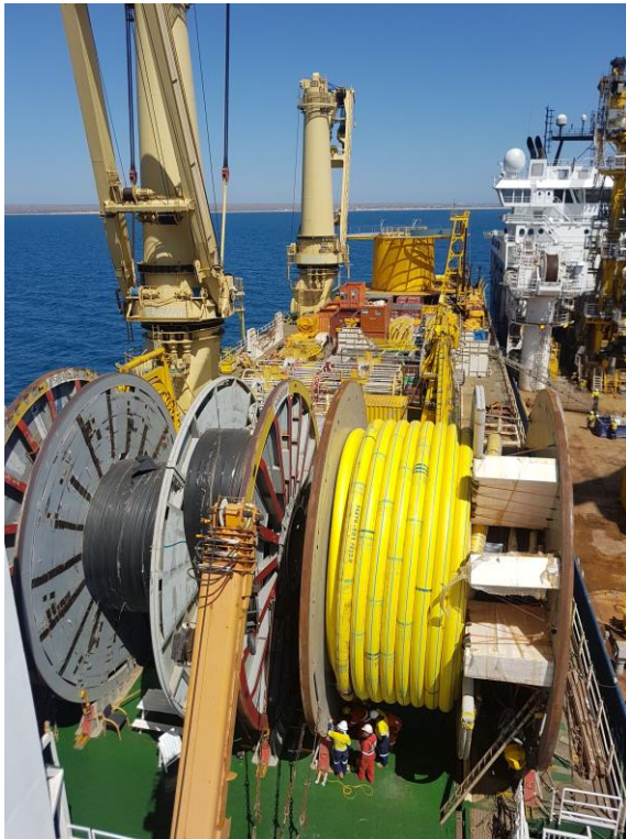
Reel on HLV next to installation vessel
