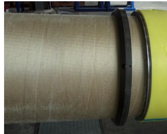
High strength tape laid on pipe
