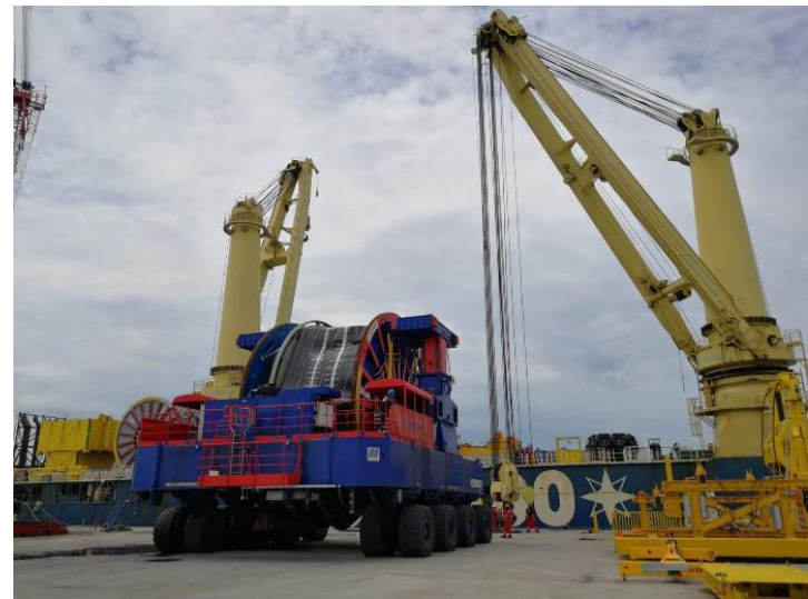
Reel transport via HLV
