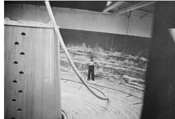
HAIS pipe (carousel lay)
