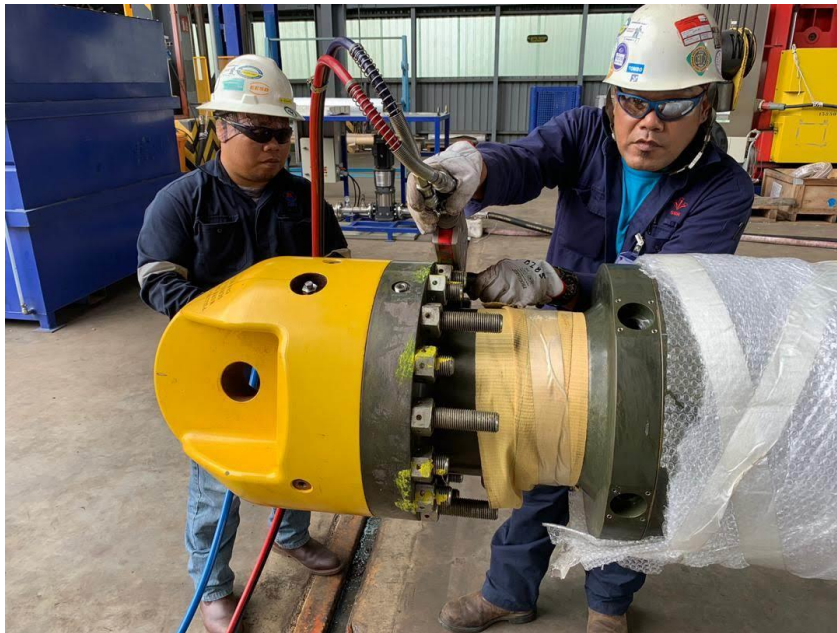
Installation of SPO (flange type) pulling head
