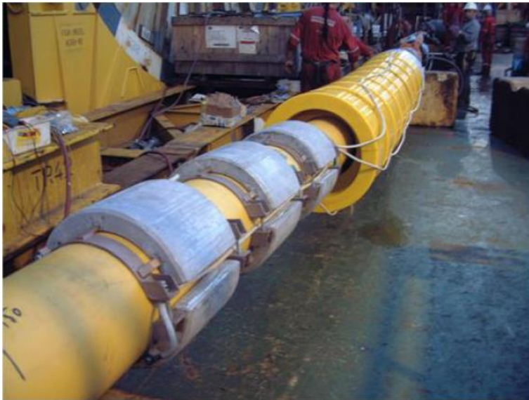
Anodes installed behind bend restrictors (note white CP cables)
