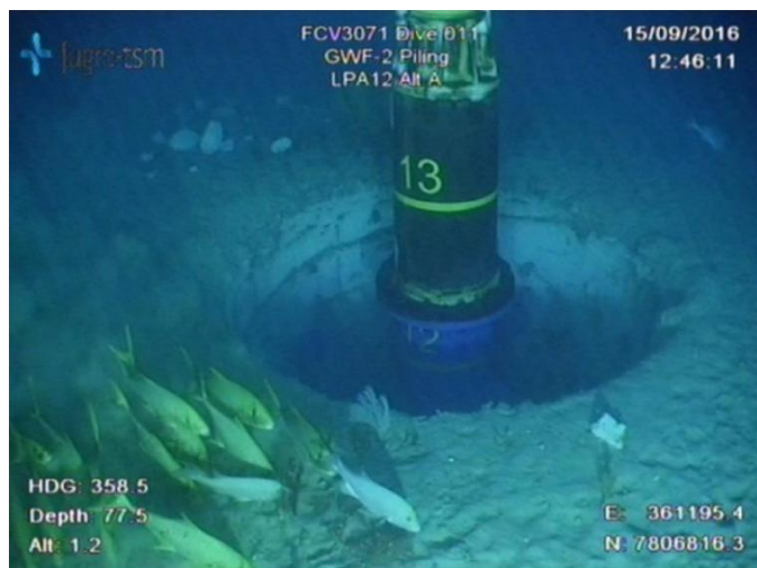
Figure 20. Visual observations of drilled hole.
