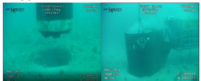
Figure 15. Pile insertion into drilled hole
