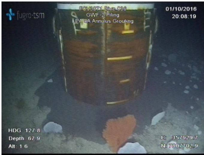
Figure 16. Grouted pile.
