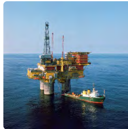
Brent Delta Topside 24,000 t Concrete
