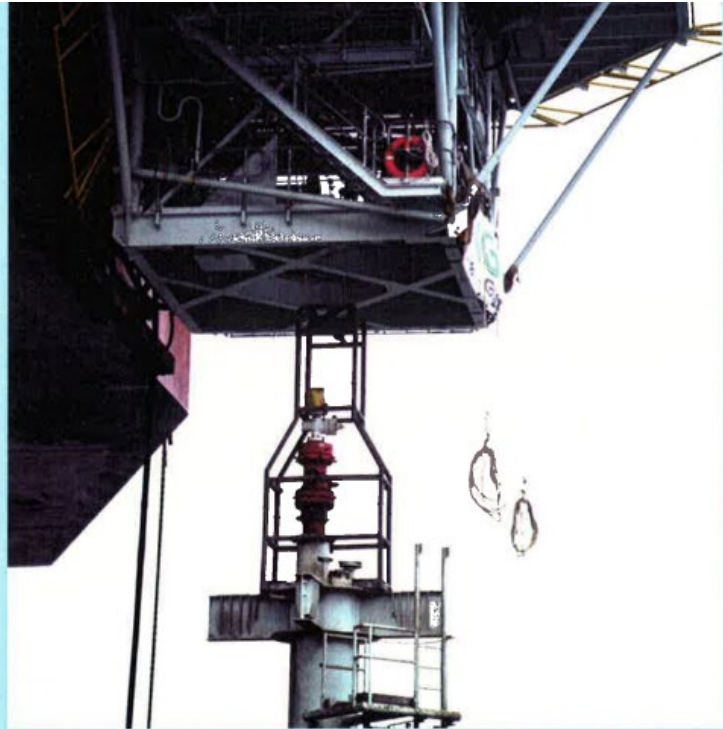
LOWERING TOPSIDES OVER WELLHEAD PROTECTION FRAME
