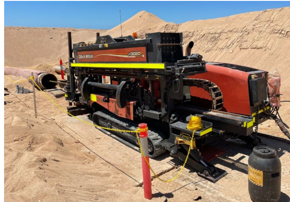
Northern – Cut & Removed from Onshore
