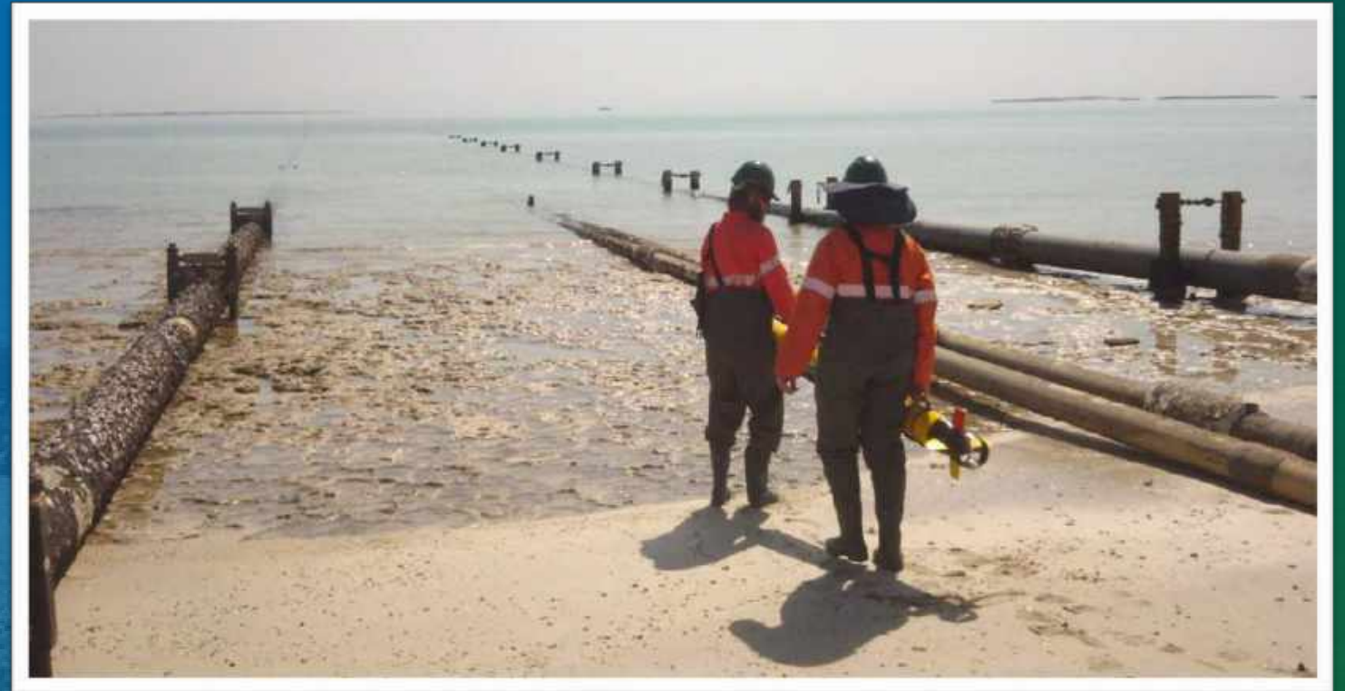
AUV DEPLOYED FROM SHORE FOR PIPELINE INSPECTION
