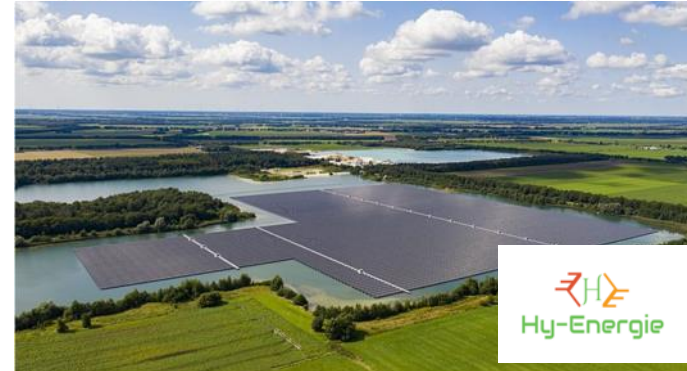
A 1.2 MW floating PV project in Hyogo Prefecture, Japan. Japan has played a leading role in the development of solutions for floating PV, as it looks to maximize generation on limited space.
