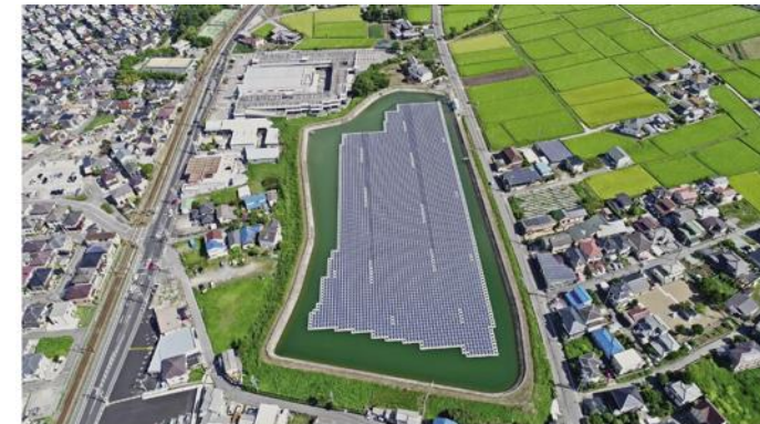
A 1.2 MW floating PV project in Hyogo Prefecture, Japan. Japan has played a leading role in the development of solutions for floating PV, as it looks to maximize generation on limited space.
